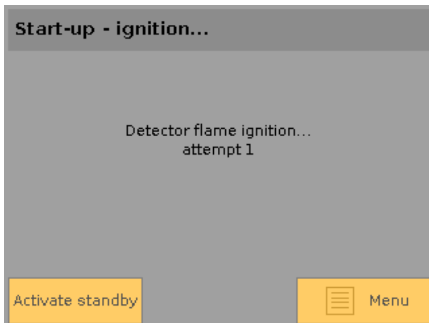
Figure 11: Ignition of detector flame
