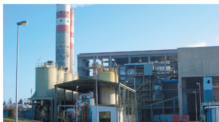
Waste Incineration Plant
