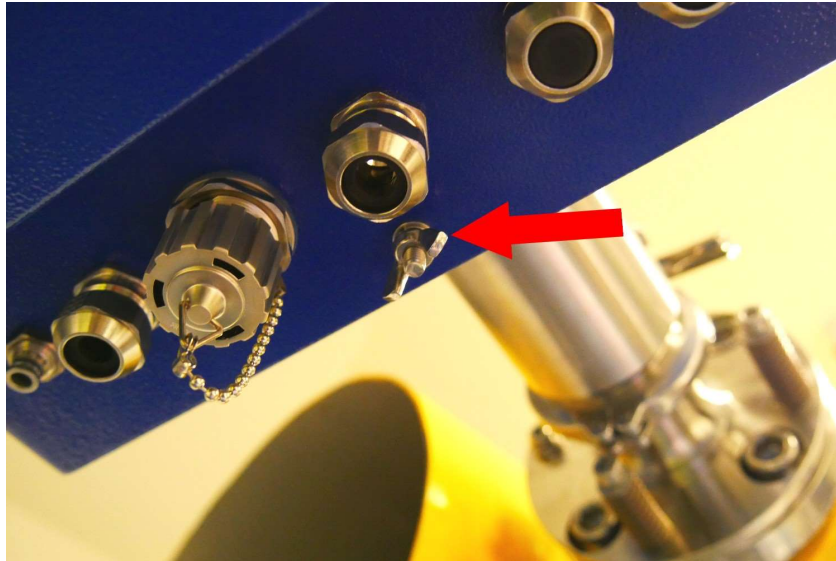
Figure 223. Grounding terminals central unit Single Gas.
