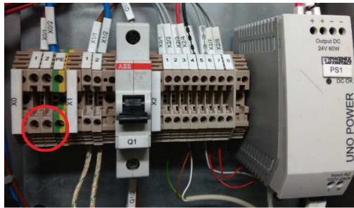
Power supply terminals block
