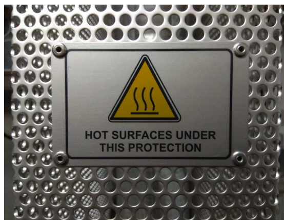
Warning indication in protection grid
